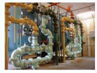
Taylor wells is filtered to remove iron and manganese caused by erosion of natural deposits in the sand and gravel aquifer. The pH of the water from the Jordan Avenue well field is adjusted using aeration to reduce the corrosivity of the water.
