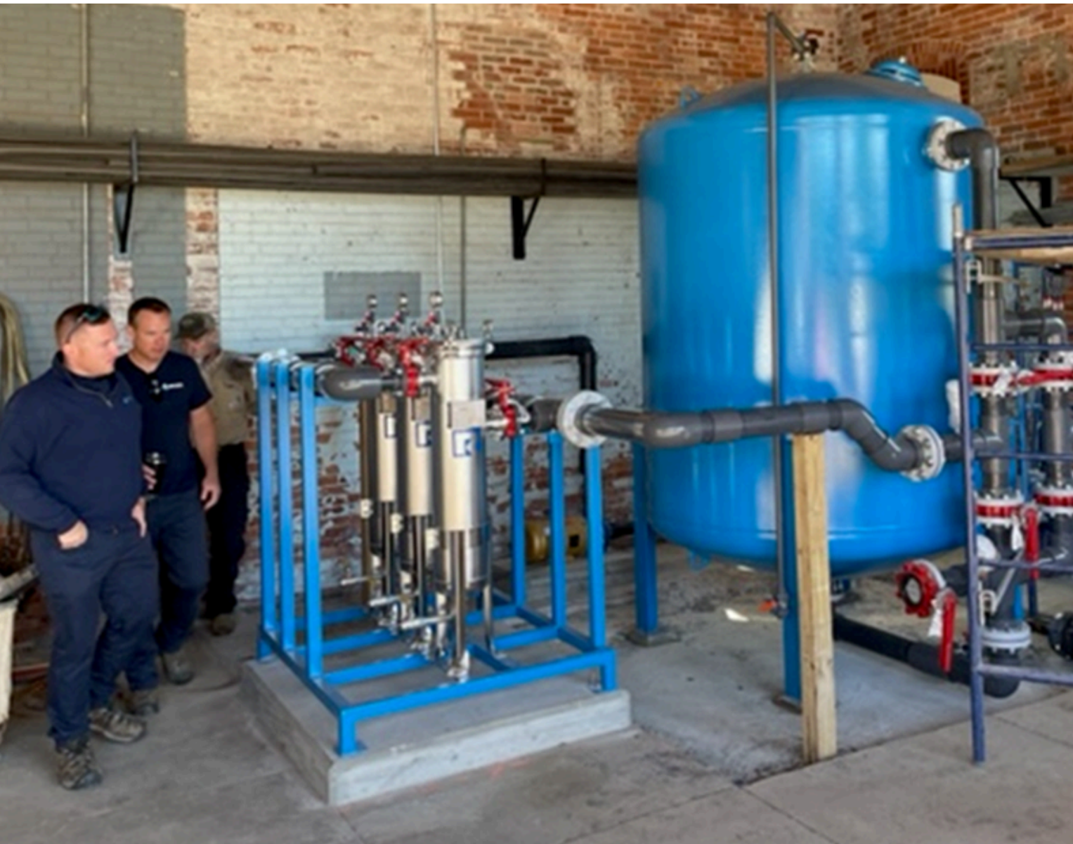
BTWD-JAS Lower Well Field PFAS Removal System. Treated water is returned to the environment.
